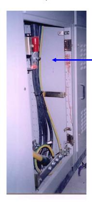
Live terminals of the 500-Amp MCCB were not covered with insulating barrier while work was being carried out at the lower compartment of the panel.
